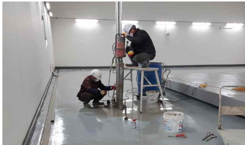
Additional penetration holes for HV of ion source
