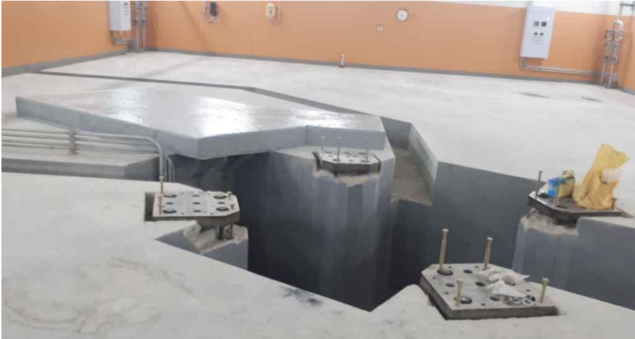
Steel plates for cyclotron support
