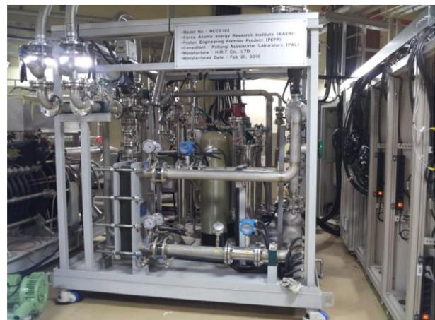
Fig. 2. Resonance frequency control cooling system
