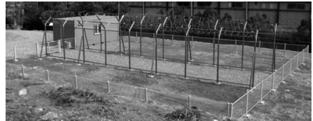
Fig. 1. Test-Bed system under construction
