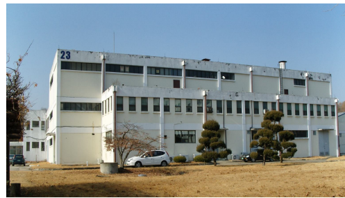
Fig. 2. Uranium Conversion Facility at KAERI.
