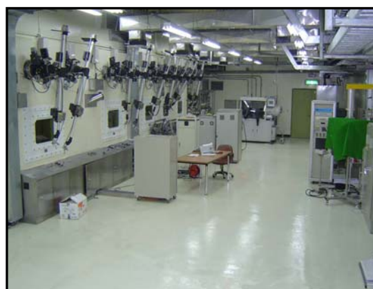
Fig. 1. The working area view of the ACPF
