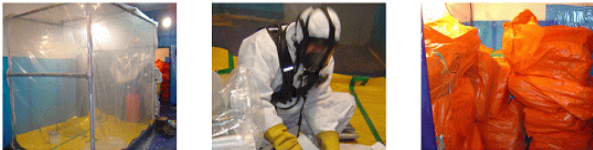
Figure 3. The preparation work for filter removal
