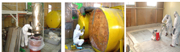
Figure 2. The liquid waste treatment facility dismantling
