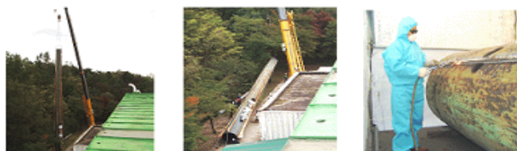
Figure 1. The stack dismantling
