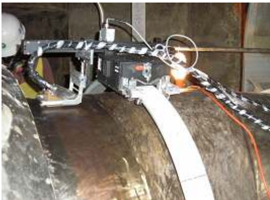
Fig 5. Field application for reactor vessel inlet nozzle of YG#1
