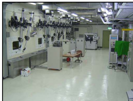
Fig. 1. The working area view of the ACPF
