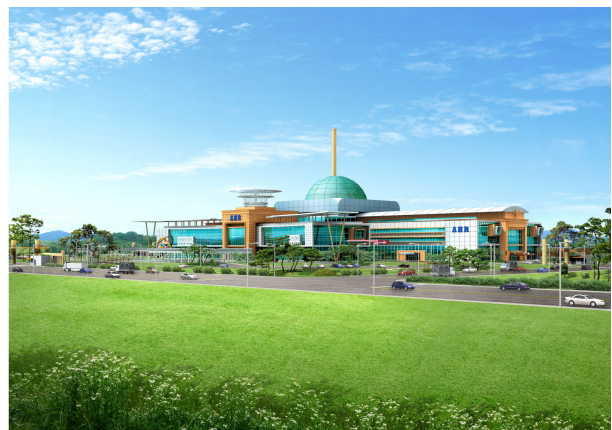
Figure 4 Right View of the AHR building and facilities
