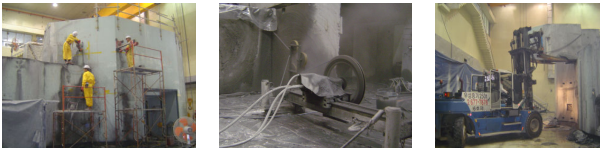
Fig. 3 Non activated concrete dismantling
