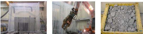
Fig. 4 Activated concrete dismantling
