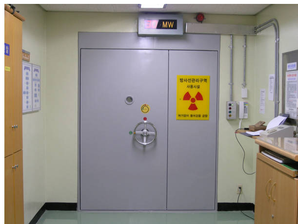
Figure 1. Security doors installed in HANARO building
