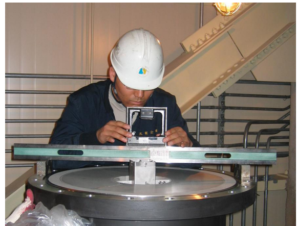
Figure 4. The vertical tolerance check of an installed section.
