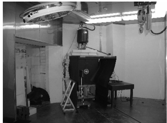
Fig.1 A view for the inside of ENF shielding room
