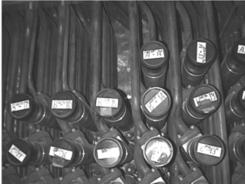
Fig.1 Feeder pipes in pressurized heavy water reactor
