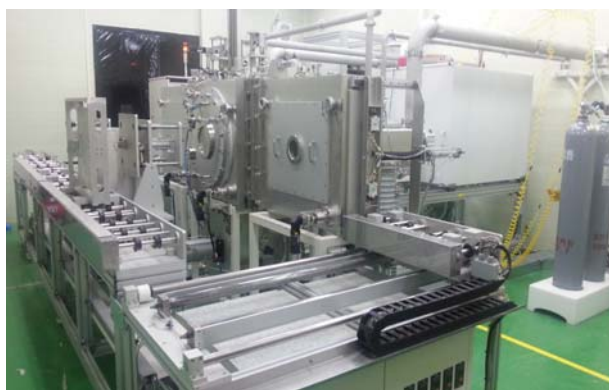
<Fig. 3. Installed ion beam facility>
