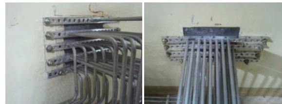
Fig. 4. Penetration Sealing work for the I&C Tubing
