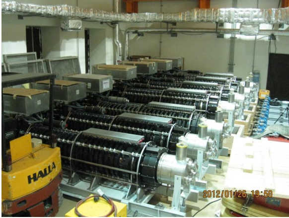
Fig. 2: 9 sets of klystron stored in the accelerator assembly room
