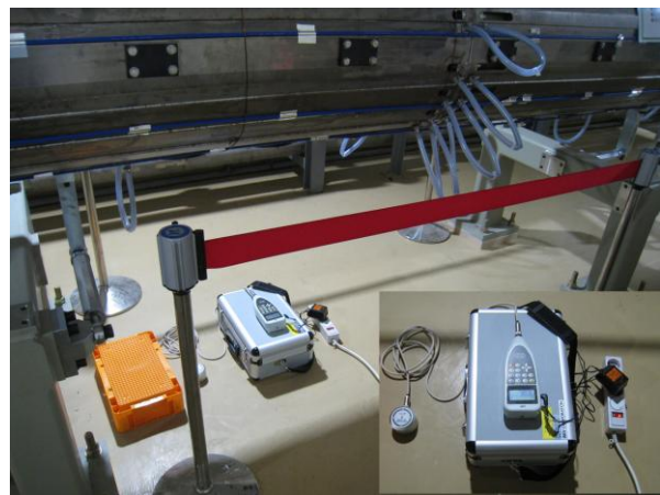
Fig. 2. Installation of vibration level meter
