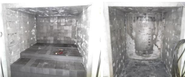
Fig.3 Dismantling of the thermal column
