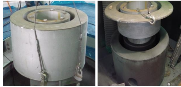
Fig.4 Dismantling of the graphite reflector
