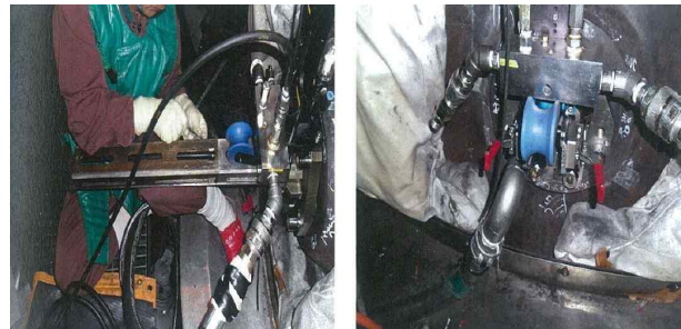
Fig.1 Installation of Lancing System at Primary Side
