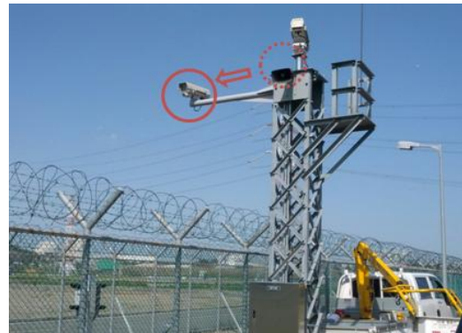
Fig.5 Usage of a bracket to cover the blind spot
