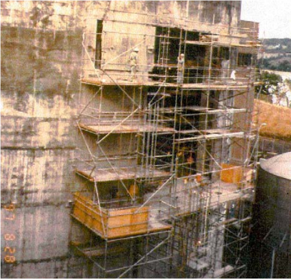
Fig. 7. Opening into Containment, Trojan.
