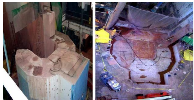
Fig 4: Diamond wire cutting of concrete block in USA
