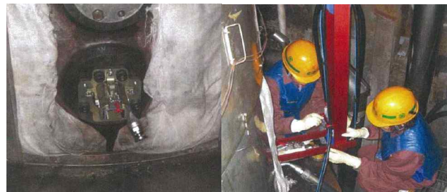
Fig.1 Installation of Lancing System at Primary Side
