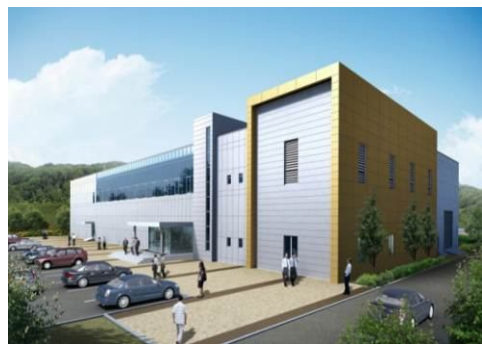
Fig. 7. Beam application research building for 1-MV ion accelerator under construction.
