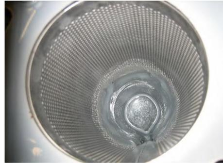
Fig. 3. Typical inside of strainer tubes after drain down
