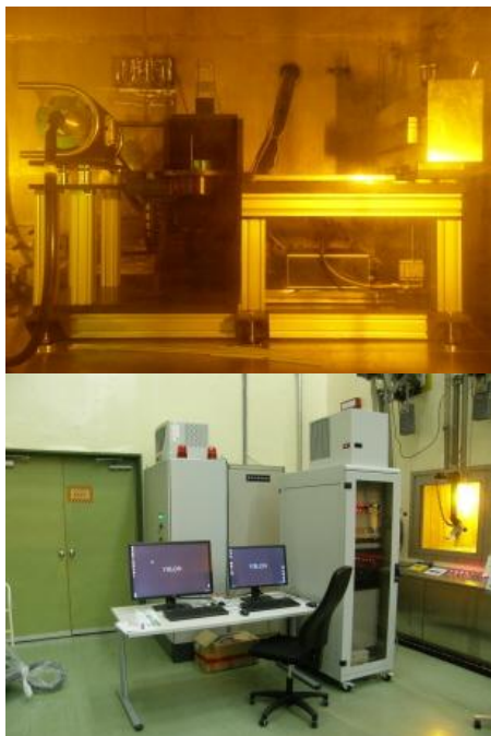
Fig.1 Installation of 450 kV X-ray
