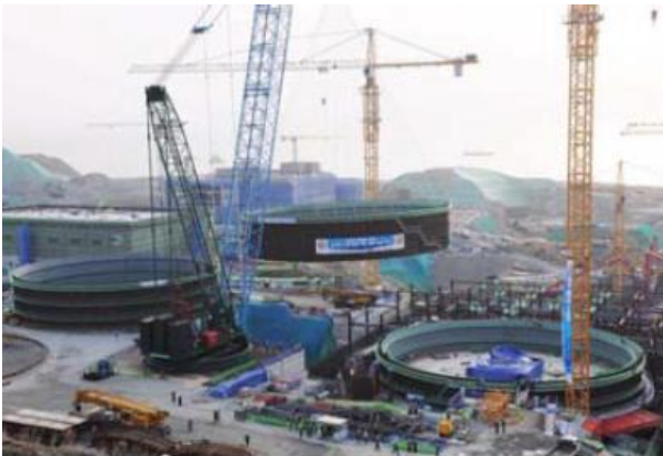
Fig. 4. Modularization of the containment liner plate assembly, Shin-wolsong 2
