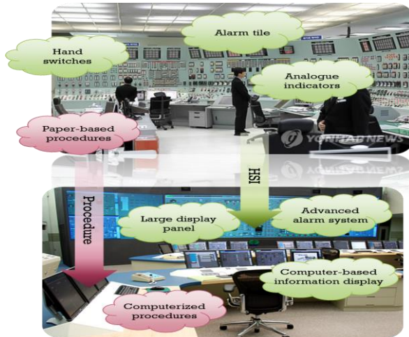
Fig. 1. Changes of control room by adopting computer-based technology in advanced MCR
