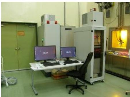
Fig. 4 X-ray controller and PLC in operating area
