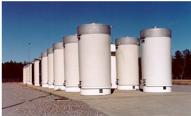
Fig. 5. CASTOR ® V/21 casks at Surry Powerstation, Virginia/USA
