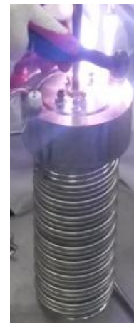
Fig.2. Welding of primary vessel.
