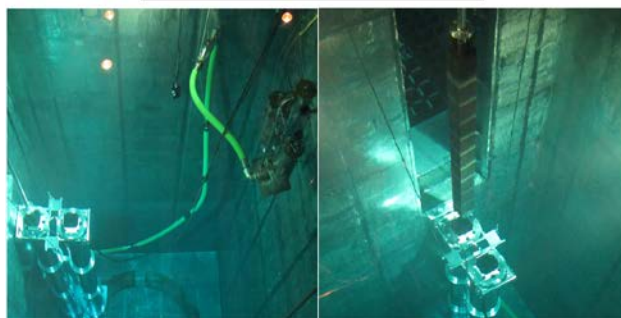
Fig 1. Outline of Crud cleaning equipment(up) and installed Crud cleaning equipment in water(down).
