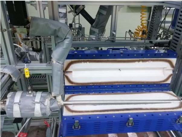
Fig. 2. Na-CO 2 mixing section equipped in the facility.
