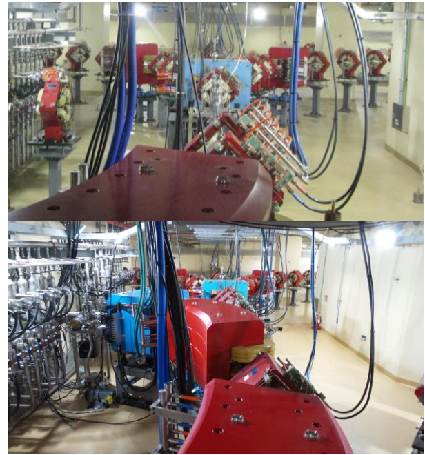
Fig. 5. Before (up) and After (down) Installation of the RI Beamline.
