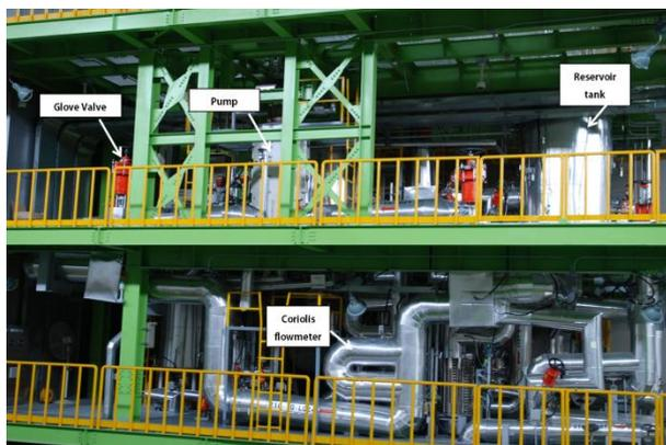
Fig. 3. Photograph of close pump performance test loop with sodium environment
