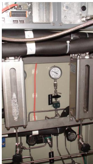
Fig. 5. Installation of drain port inside the sampling panel for gas
