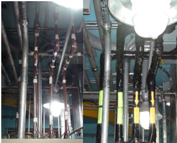
Fig. 3. Installation of heating cable and heat insulating material
