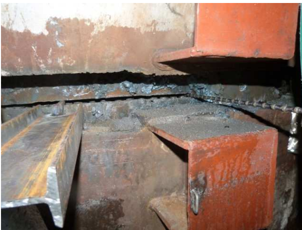
Fig.4. Steam Generator cutting under TSP-1
