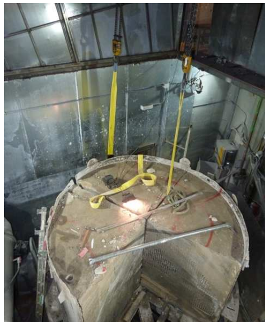
Fig.5. Steam Generator top set after concrete, cut and first part removal
