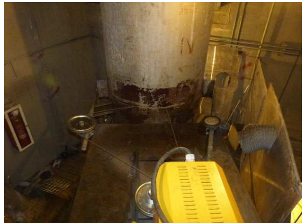
Fig.2. Pressurizer cutting
