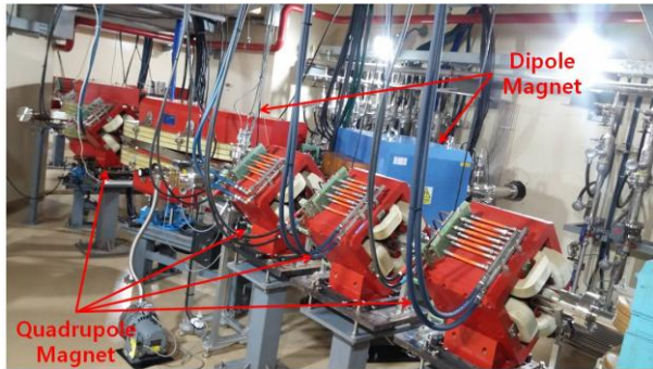
Fig. 3. Installation and alignment of magnets
