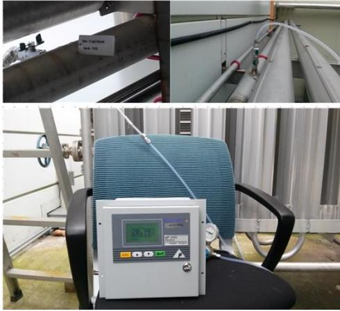
Fig 4. Oxygen sensor connected to PSV102 valve
