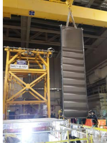
Fig. 5. Installation of pool door
