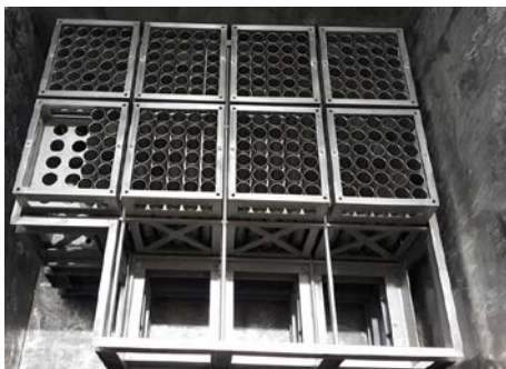
Fig. 5. Installation of spent fuel storage rack
