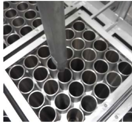
Fig. 2. Spent fuel storage rack and dummy fuel assembly
