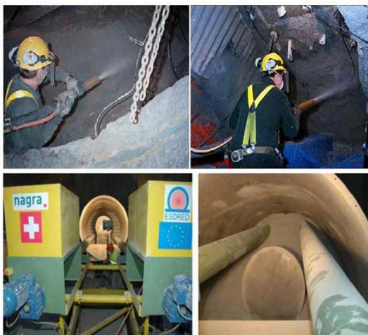
Fig. 4. Gap-fill installation technologies: shotcrete-blowing method (upper) and twin auger method (bottom).
