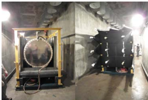
Fig. 2. NEOS detector installation in Tendon gallery at Hanbit power station unit 5.
