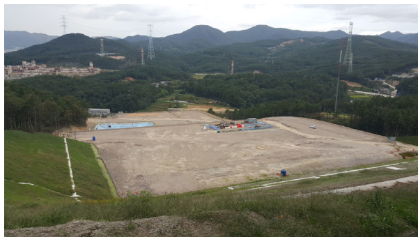
Fig. 1. Site grading work.
