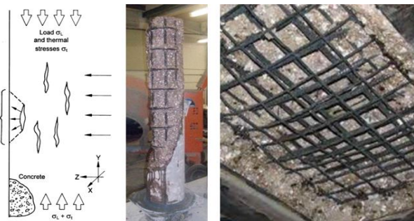
Fig. 13. Spalling failure mechanism of concrete and concrete failures on column and slab by spalling during fire
