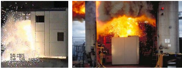
Fig. 5. Cabinet fire due to high energy arc faults (HEAF)
