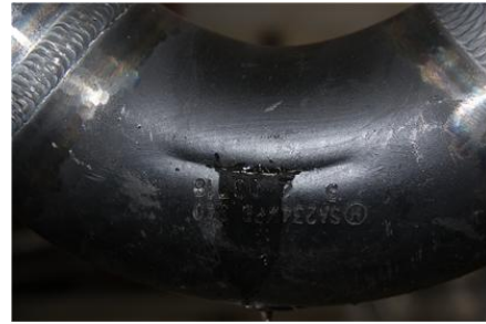
Fig. 5. Ultimate failure state of elbow specimen: penetration crack & leakage of water at the crown of elbow.
