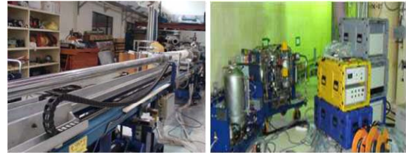
Fig. 6 HDM Mock-up and Installation in Reactor Building
