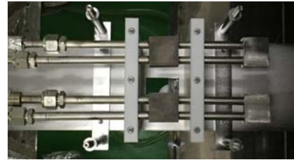
Fig. 1. Fabrication and installation of W HIP joining mockups
