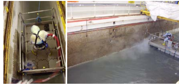
Fig. 1. Ultra-high pressure washing of the Bradwell pond.
